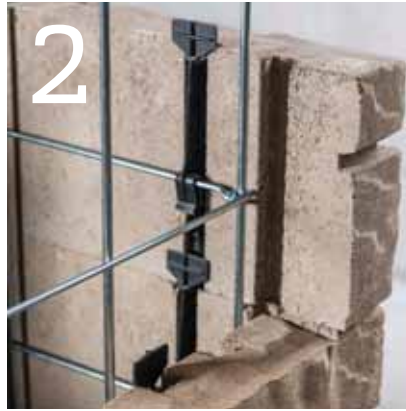
2 Use connector to attach Tandem Units to grid
